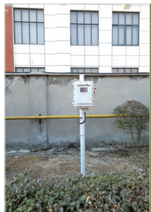
Air VOC monitoring equipment installed on site
